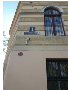
External video surveillance of the 3rd building
