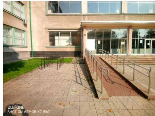
Ramp and bicycle parking near the educational building №1 at 2/4 Karpinskoho Street
