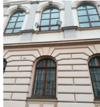
LED lighting (main building, Lviv)
