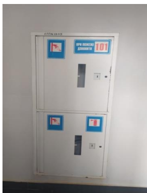
The fire shield of the 23rd building
